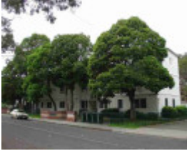
princes hill solly avenue princes hill solly avenue 21
