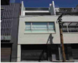
richmond wangaratta street richmond wangaratta street 28
