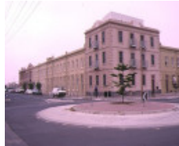
1 former swallow & ariell biscuit factory stokes street port melb corner building jun1995
