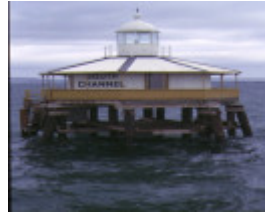
1 south channel pile light light after relocation front view
