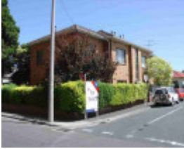
richmond woodlawn street richmond woodlawn street 12-14
