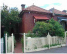
carlton north station street carlton north station street 447
