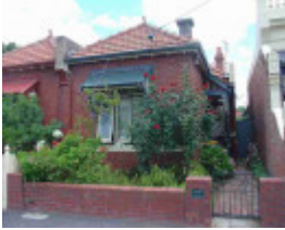
carlton north station street carlton north station street 449
