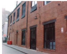
Former Angliss Stables May 2003
