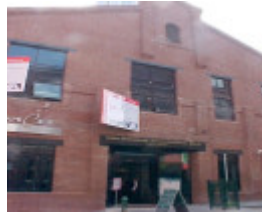
Former Angliss Stables May 2003
