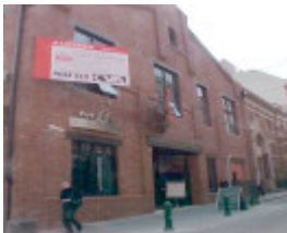
Former Angliss Stables May 2003
