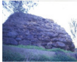
h00389 portarlington mill turner crt portarlington remains of rear boiler house she project 2003
