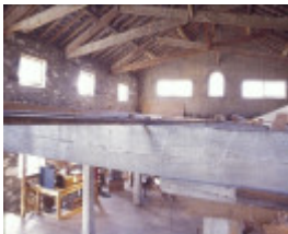
h00389 portarlington mill turner crt portarlington top floor north end she project 2003
