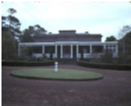
1 maretimo portland front view of house
