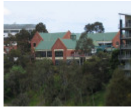
Rear 64-78 Trenerry Crescent.jpg
