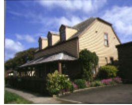
1 former steampacker hotel front view
