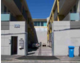
fitzroy argyle street fitzroy argyle street 190
