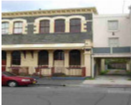
National School - 40 Bell Street
