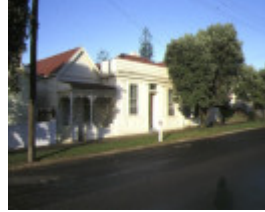
1 former builders inn portland street view aug1985
