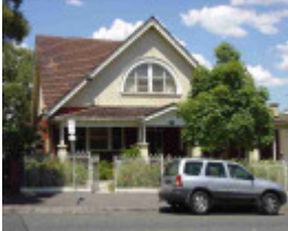
richmond docker street richmond docker street 25-27
