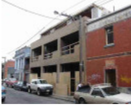
fitzroy argyle street fitzroy argyle street 30-34
