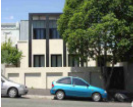
richmond docker street richmond docker street 33
