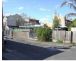
Fitzroy John Street 21-23 REAR CREMORNE Street FACADE.JPG
