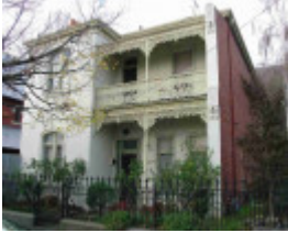
Fitzroy George Street 268 Residence.JPG
