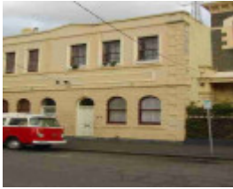
National School - 44 Bell Street
