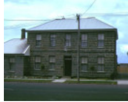
1 victoria house portland front view jan1994
