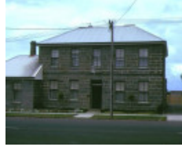
1 victoria house portland front view jan1994
