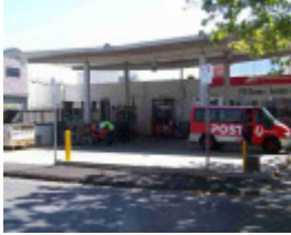
fitzroy argyle street fitzroy argyle street 201
