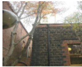
Prahran Town Hall NW Rear Corner of First Town Hall May 05
