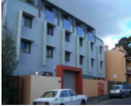
fitzroy fitzroy street fitzroy fitzroy street 128
