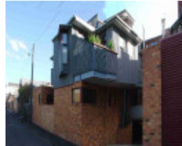
Fitzroy George Street 58-62 rear.JPG
