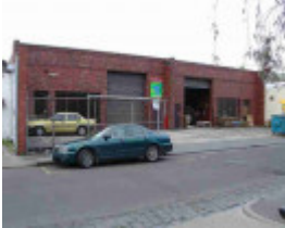
fitzroy argyle street fitzroy argyle street 51-53
