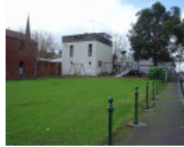
Fitzroy George Street 227 rear.JPG
