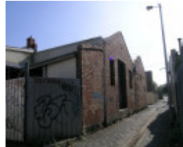
Rear of 428 Brunswick Street.JPG
