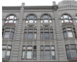
Elaborate detailing on the eastern face
