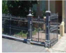
Fence - 419 Canning Street
