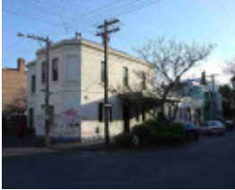
fitzroy moor street 74
