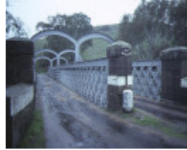
1 Redesdale Bridge redesdale end of bridge
