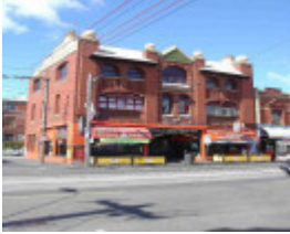
Fitzroy Brunswick Street 320-322.JPG
