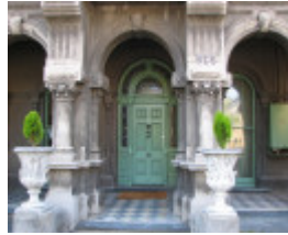
FORMER LALOR HOUSE SOHE 2008
