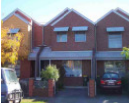
fitzroy north bennett street fitzroy north bennett street 99
