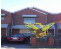
fitzroy north bennett street fitzroy north bennett street 101
