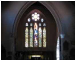
ST STEPHENS ANGLICAN CHURCH SOHE 2008
