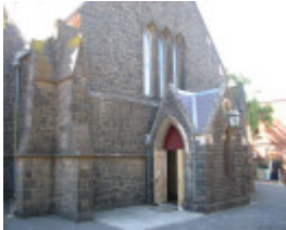
ST STEPHENS ANGLICAN CHURCH SOHE 2008
