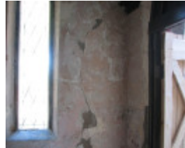
ST STEPHENS ANGLICAN CHURCH SOHE 2008
