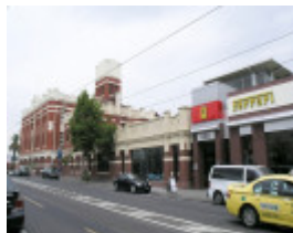
FORMER BRYANT & MAY INDUSTRIAL COMPLEX SOHE 2008
