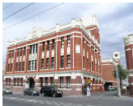
FORMER BRYANT & MAY INDUSTRIAL COMPLEX SOHE 2008
