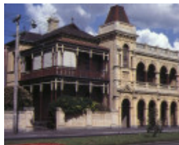
1 urbrae hoddle street richmond front view
