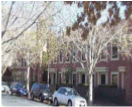
Cable Tram Engine House - 1015 Rathdowne
