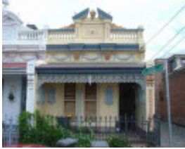
carlton north richardson street carlton north richardson street 89
