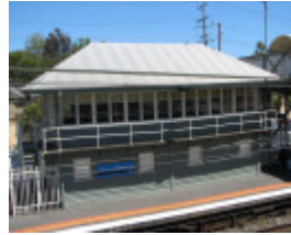
RINGWOOD RAILWAY STATION SOHE 2008
