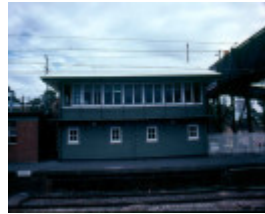
Ringwood Railway Station Railway Signal Box
