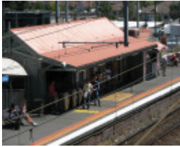
RINGWOOD RAILWAY STATION SOHE 2008
