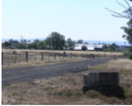
DEANSIDE WOOLSHED COMPLEX SOHE 2008
