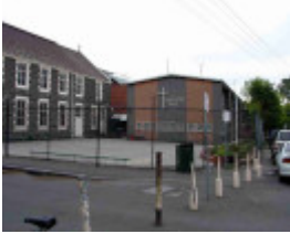
Fitzroy King William Street 97-107 School.JPG
