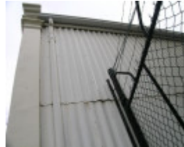
All Saints Iron Hall - side wall
