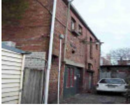
fitzroy north bakehouse lane fitzroy north bakehouse lane 1
