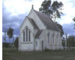
h00599 1 st marks anglican church cnr albert hood streets rosedale rear view church sep1983
