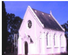
St Marks Anglican Church Albert St Rosedale North West Profile
