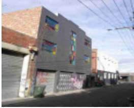
fitzroy little smith street fitzroy little smith street 91
