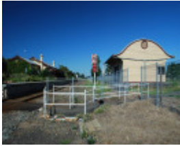
ROSEDALE RAILWAY STATION COMPLEX SOHE 2008
